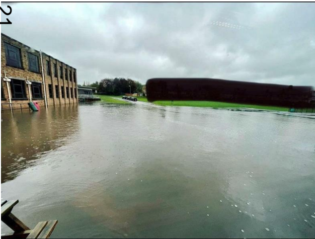
Figure 11: Flooding experienced in Flintshire School.
